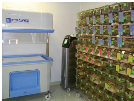
Figure 2. Nude mice are maintained in a separate room with an IVC system and air handling unit.
